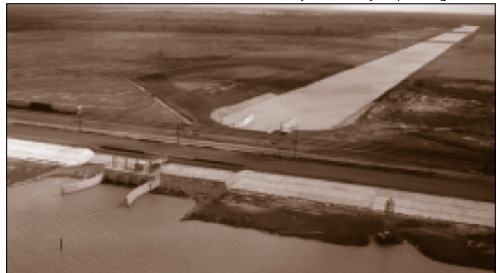
Davis Pond freshwater diversion structure. Photo courtesy of U.S. Army Corps of Engineers.
