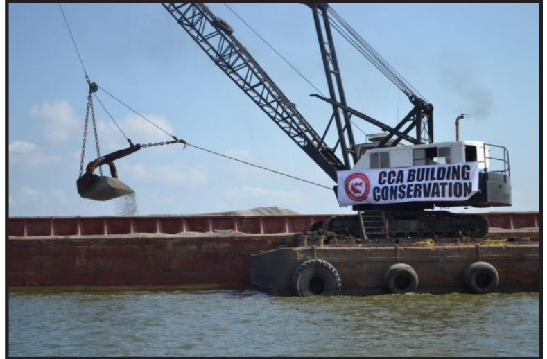
Construction on the Reef. Photo credit: Louisiana Department of Wildlife and Fisheries
